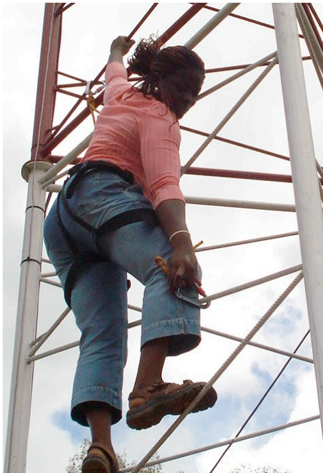
Figure 11.3: Omolayo Samuel, one of the staff of Zittnet, does not fear the height of the 45m tall tower as she is aligning the antennas hosted in the top of the tower.
