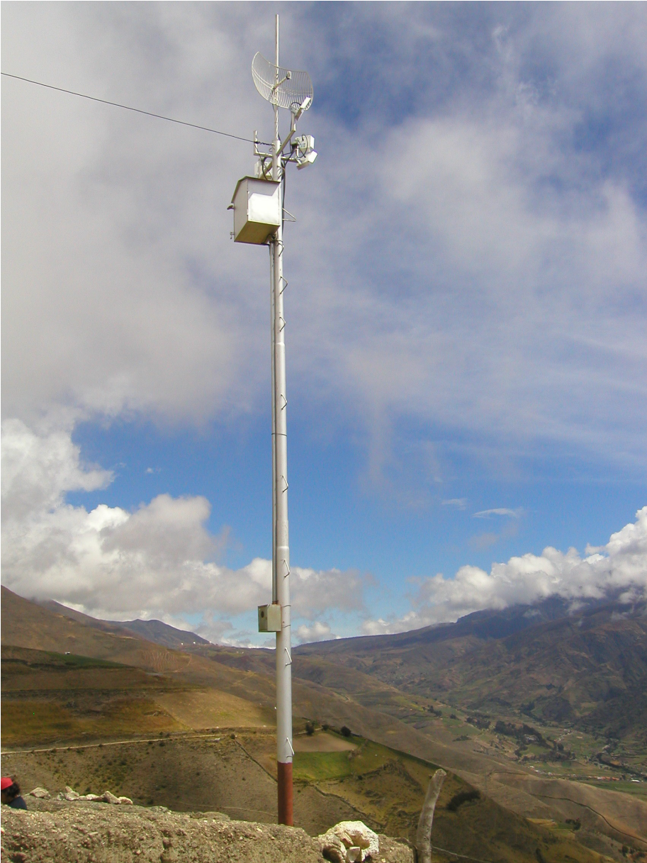
Figure 8.3: A simple self-supporting tower.
