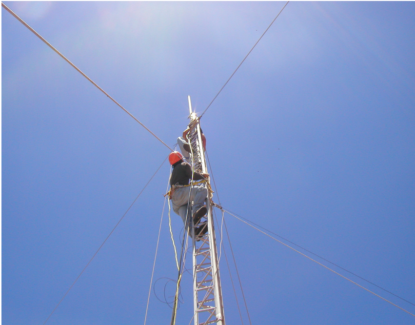
Figure 8.2: A climbable guyed tower.
