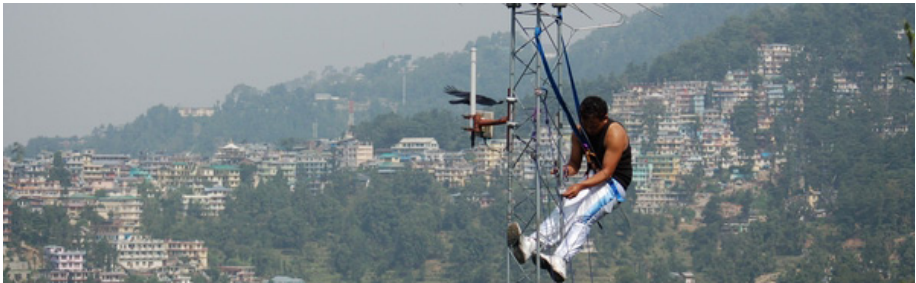
Figure 11.5: Dharamsala installer working on a tower
