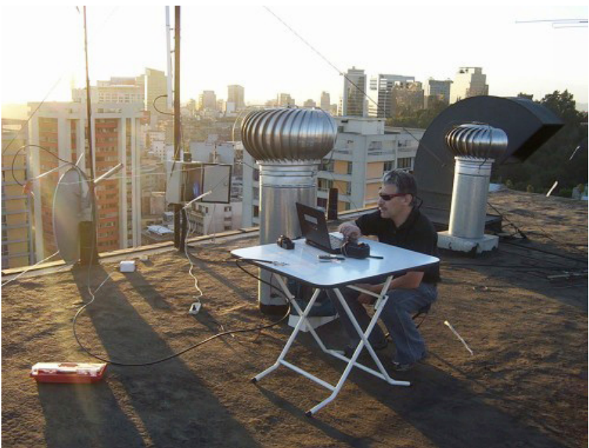
Figure 11.23: Downtown node connected to the Santiago southern node. Note the parabolic antenna for backhaul and the slotted antenna to connect the clients.
