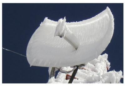
parabolic grid (covered by snow)
